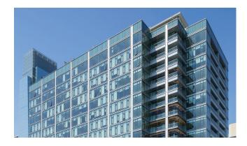
With a collaborative team, high-performance glazing system and the owner's approval, Franklin Tower transformed from concrete offices to an attractive, glass-clad, energy-efficient residential high-rise in six months.
