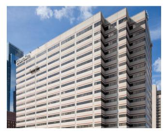
Prior to its transformation, the building served as an office tower since the 1980s with an aging facade of precast concrete and single-glazed strip windows.
