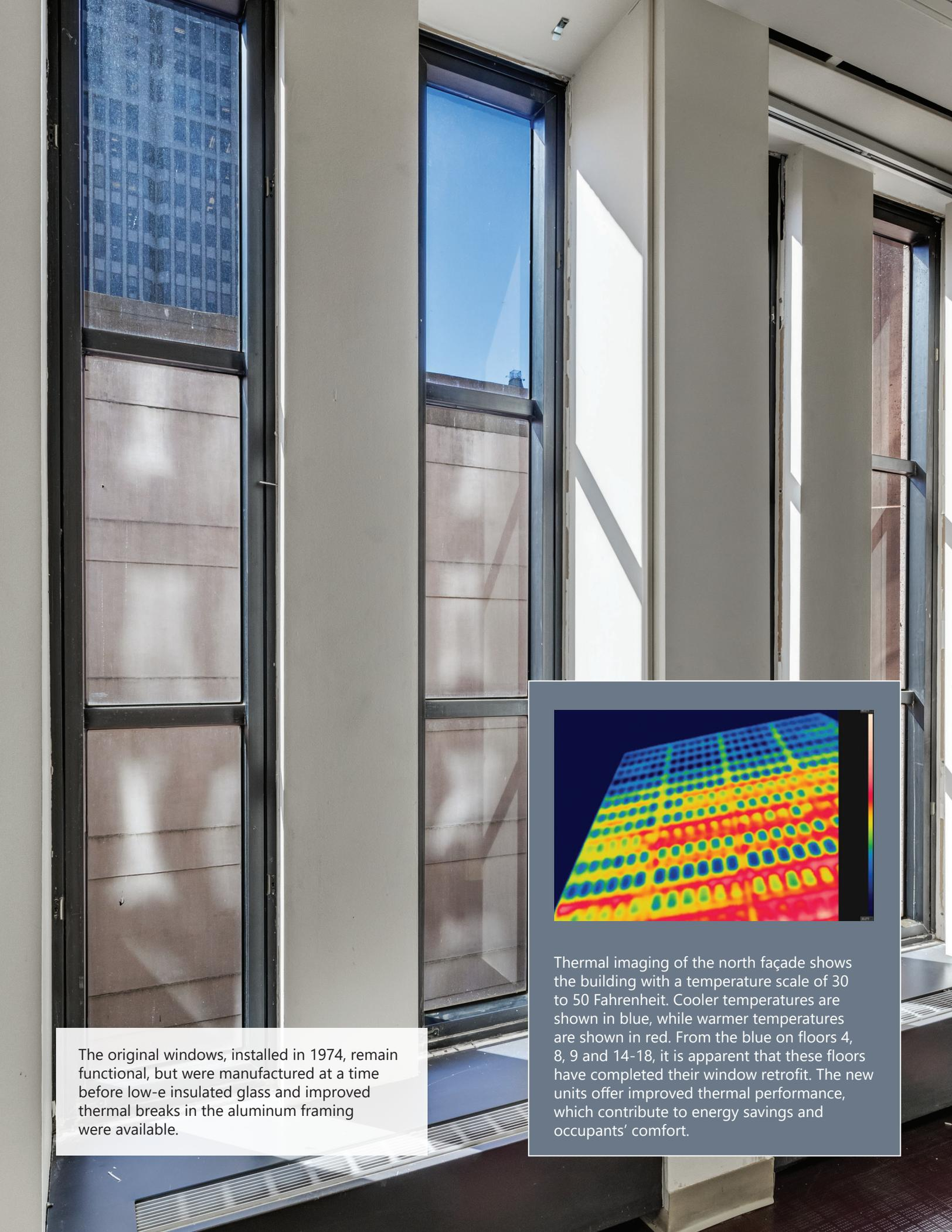
The original windows, installed in 1974, remain functional, but were manufactured at a time before low-e insulated glass and improved thermal breaks in the aluminum framing were available.
